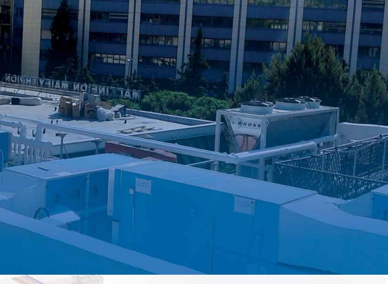
EXP Systems is the multi-purpose ecological system designed by Rhoss to meet cold and hot water demands simultaneously or independently with a single unit. It is designed for use in 2, 4 and 6-pipe systems, any time of the year.
