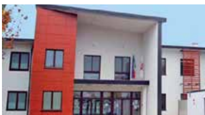
New Italo Calvino School Via di Santa Maria a Cintoia, 8 (FLORENCE) - ITALY
